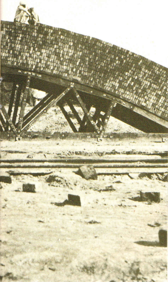
section to be moved bodily on tramrails.
