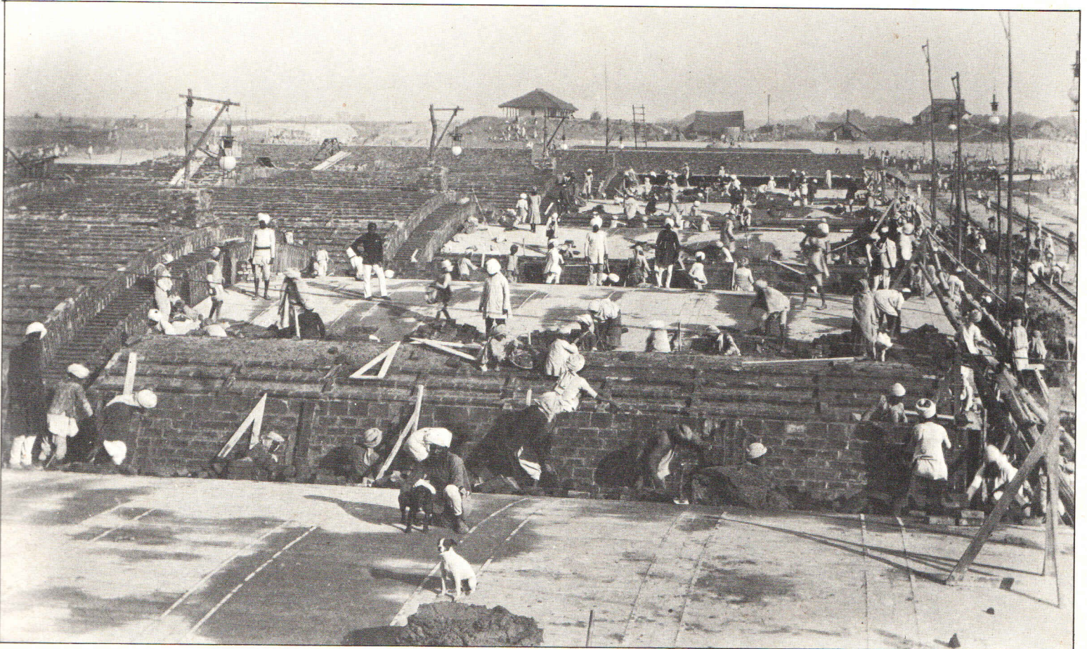
Workmen swarm busily over the half-completed arches of the Nadri Aqueduct, laying some of the 58 million bricks it took to complete them.
