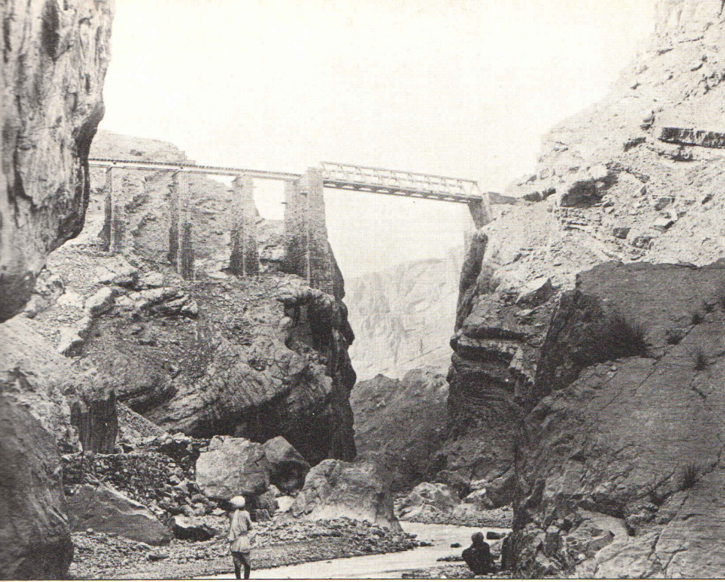
The Chappar Rift railway bridge, 233 feet above the ravine, was part of the line that was virtually the only way into the hostile lands on the southern borders of Afghanistan.
